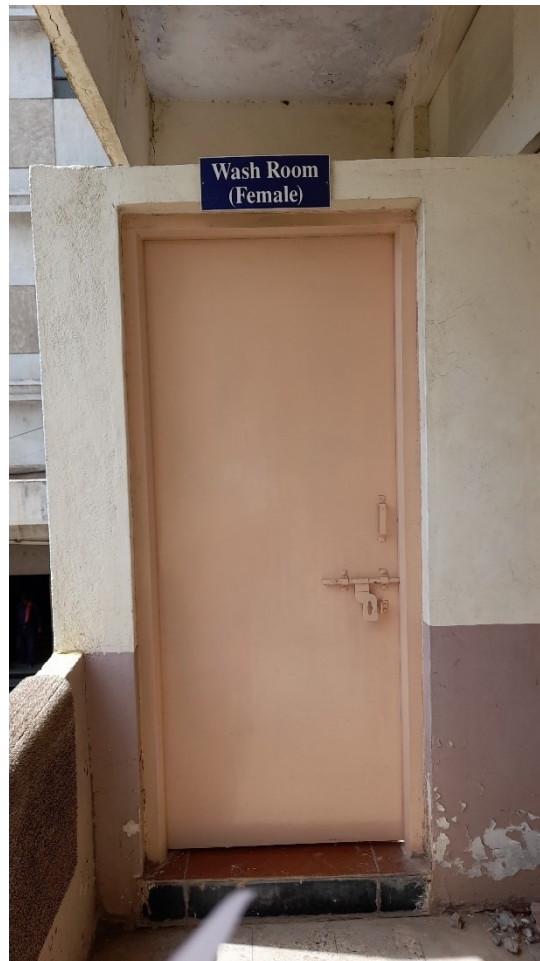
Ladies Wash Room
